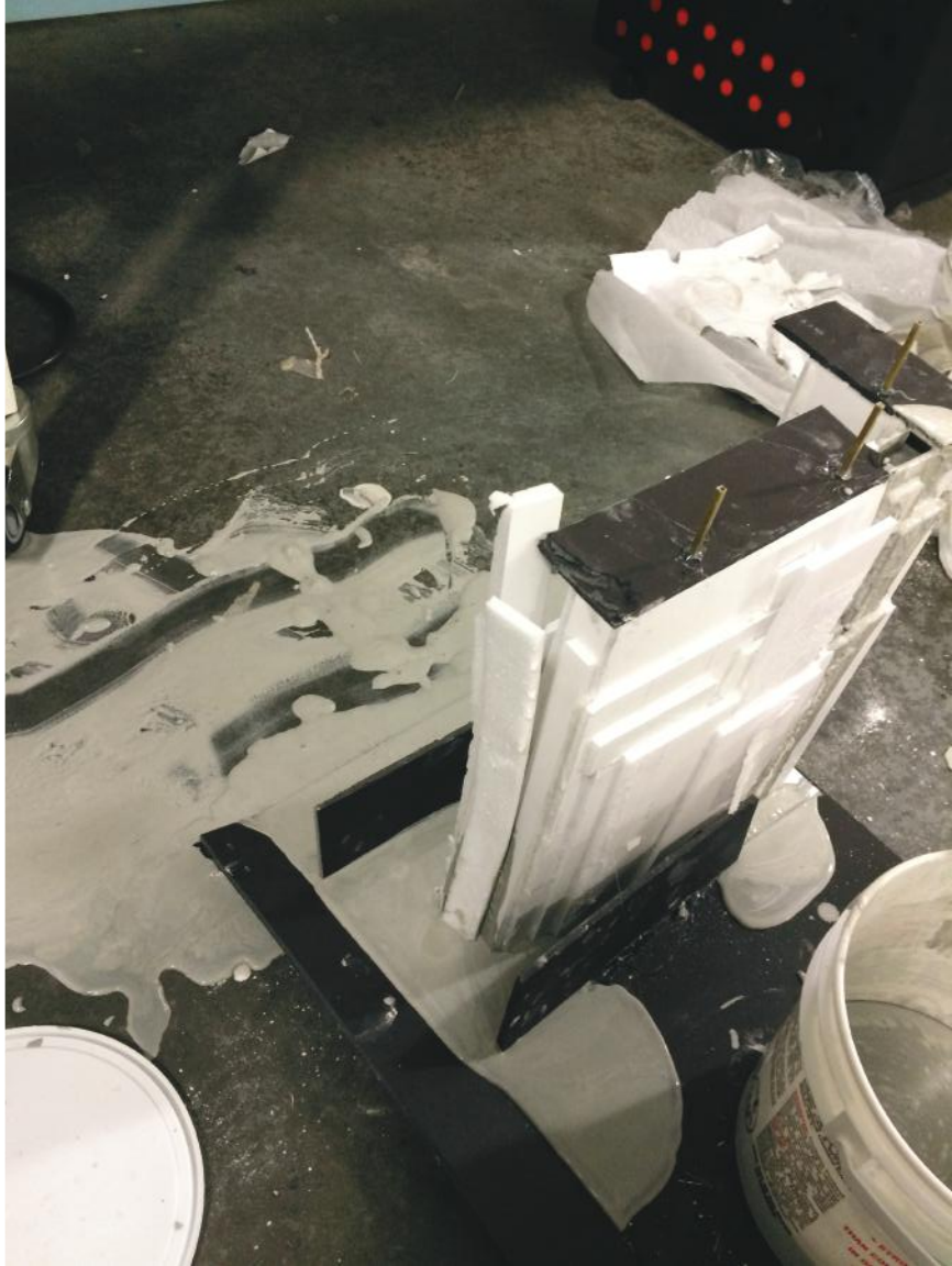
some leakage but with success
